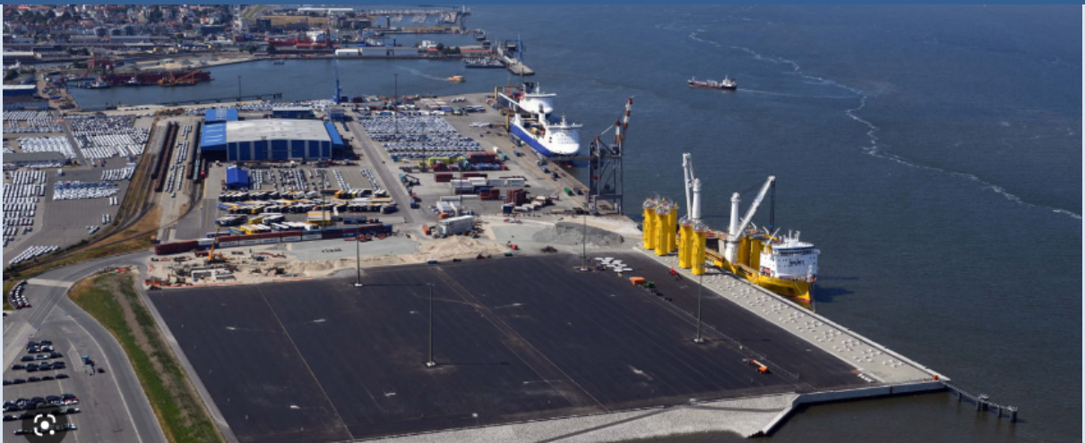
Figure 10-5: Cuxhaven Deepwater Berth [51]
