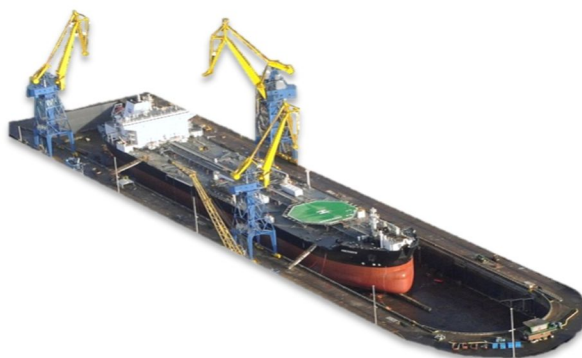
Figure 8-6: Ship Repair Drydock and Craneage
