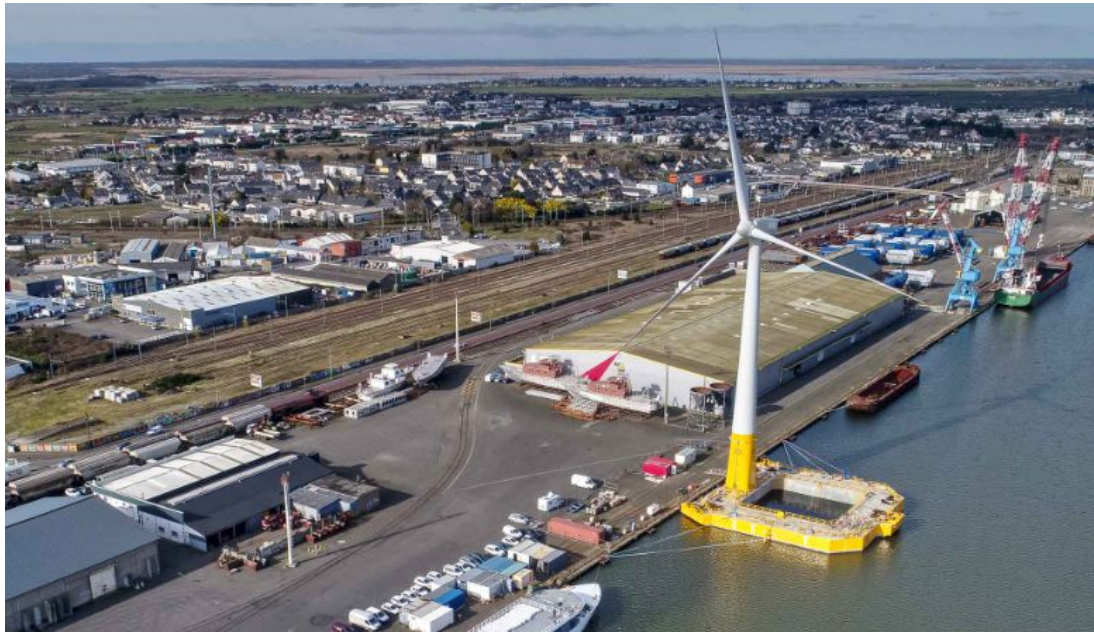
Figure 2-7: Floatgen Demonstrator with Barge unit at Quayside in Saint-Nazaire [19]
