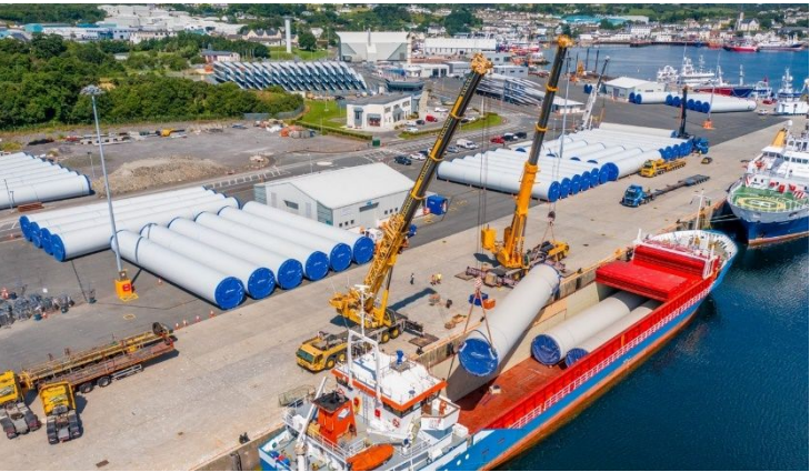
Figure 8-24: Killybegs Quayside Handling Onshore WTG Towers
