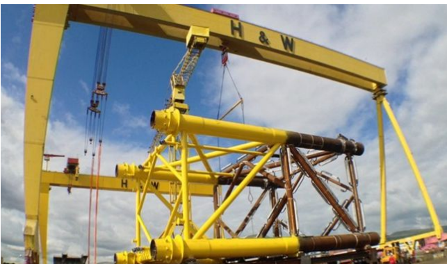
Figure 8-5: Humber Gateway Substation Jacket Lifted by H&W Gantry Crane
