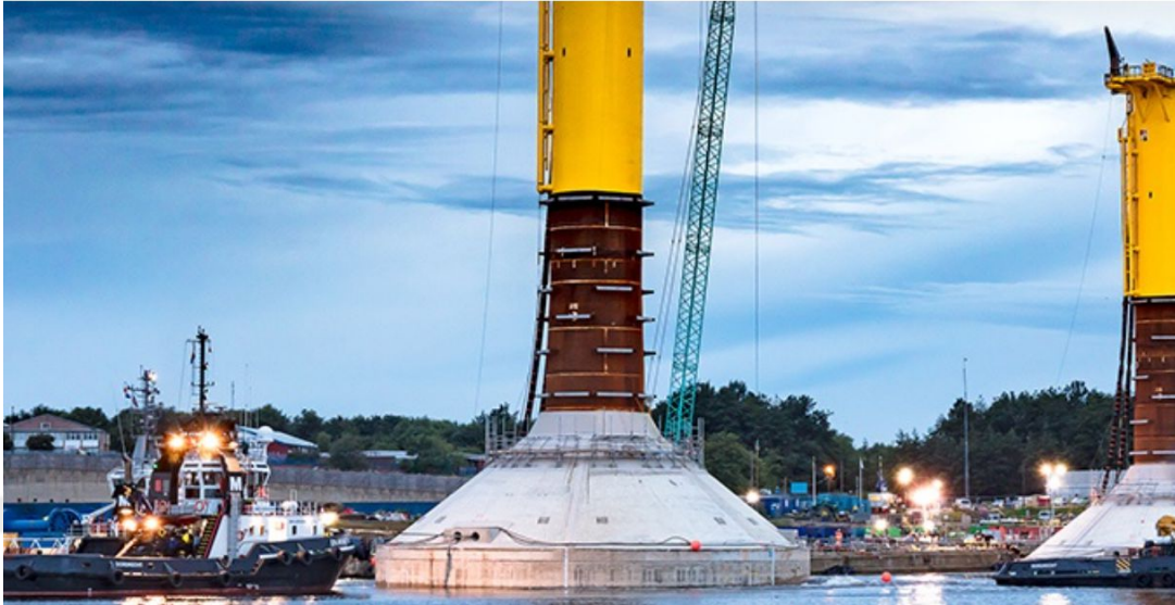
Figure 2-3: Gravity Foundations for Blyth Offshore Wind Farm [11]
