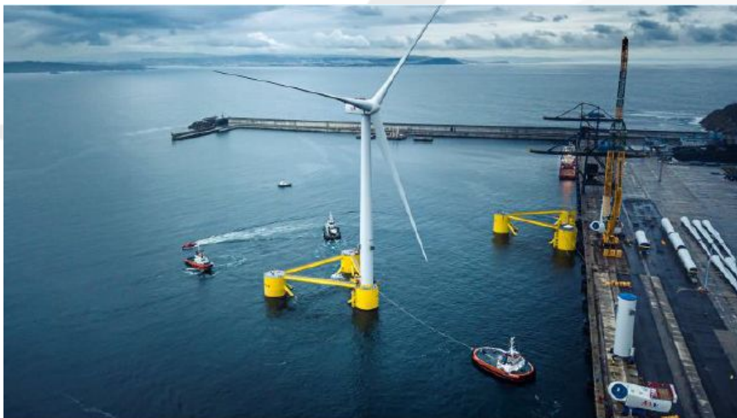
Figure 2-6: WindFloat Atlantic in Portugal with Semi-Submersible unit at Quayside in Ferrol, Spain [18]
